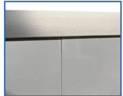
Close Up View of Butt Seam
